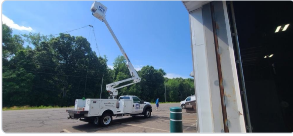
Figure 1: Marcus Radio utility boom truck staged on site during initial preparations.
