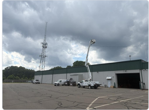
Figure 2: Site overview showing proximity to communications tower and warehouse infrastructure.
