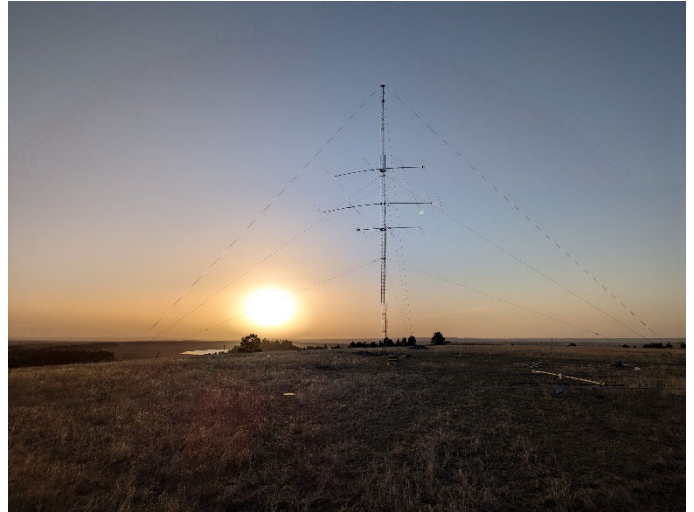
The KM7W station is high on a hill in central Montana, to the point that antenna-planning software HFTA says any tower above 100 feet is a waste of steel. (Chris Hurlbut, KL9A, photo)
