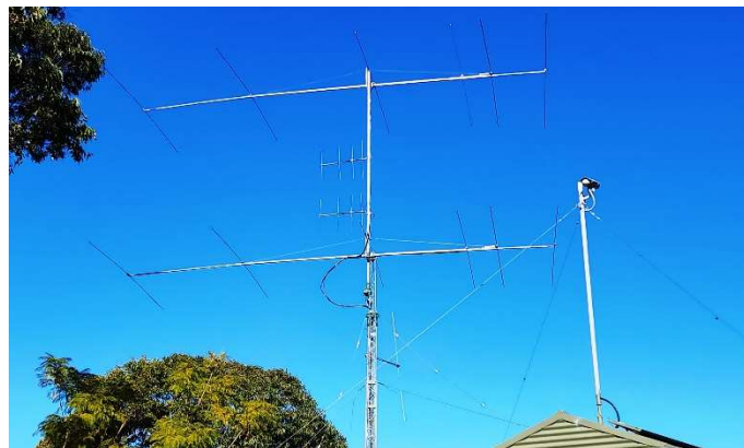
The stack of 6-element OWA Yagis at VJ2J [David Burger, VK2CZ photo]
