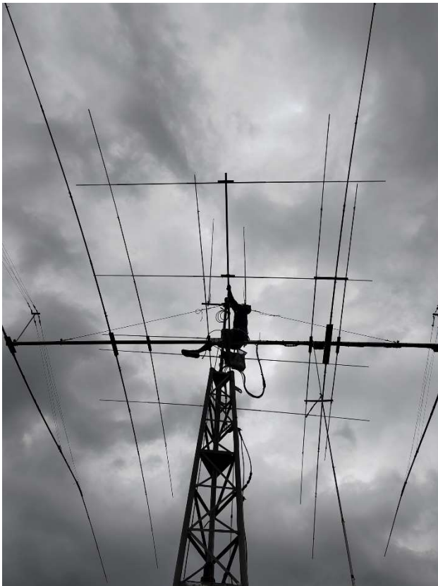
Ian, 4F1EBD installing his 5-element beam before the start of the contest. [Ian Uy, 4F1EBD, photo]
