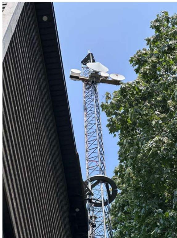
Kevin, VE3KH, rebuilt his antenna system in 2023 with a rotating tower and dish-mounted gear for all bands from 10-78 GHz. His lakeshore location in FN03cg is centrally located for activity and his signal is always strong, earning him the nickname "Mr Reliable." (At least that's what I call him.--K2UA) (VE3KH photo)
