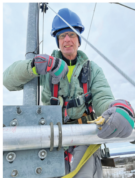
Ron Schwartz, VE3VN, installed a new three-element 40-meter Yagi at 150 feet on his tower, in preparation for ARRL November CW Sweepstakes. Ron took first place in Canada in the Single Operator, QRP category. [Ron Schwartz, VE3VN, photo]
