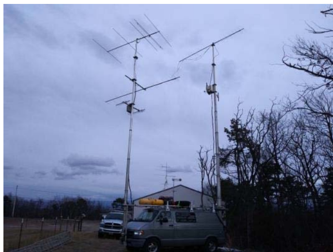
The antenna farm used at K8GP. Note the K8GP rover vehicle antennas and masts used for fixed operation. (Photo K1RA)
