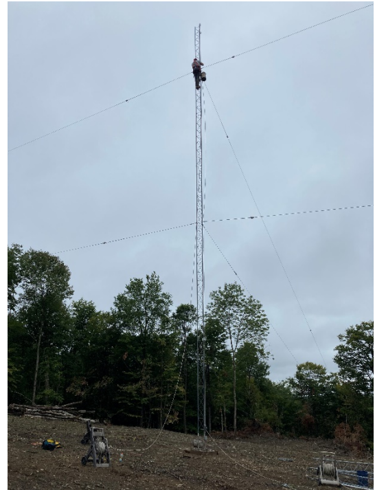
AB3CX's 160-meter vertical being assembled and installed by Ray, W2RE. Photo courtesy of AB3CX]
