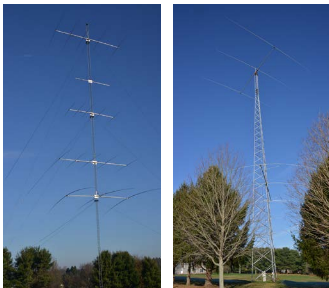
WZ8P's station and antennas. Having 3 separate 3L 40m yagis and 4 different 80m antennas from dipoles to 4L wire beams, sure helps the ERP situation when operating QRP! (Photos courtesy of WZ8P)
