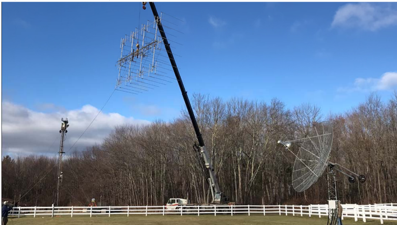
The 48 Yagi 432MHz array at Frank NC1I's QTH was removed in 2019 as pictured above and rebuilt for this year's ARRL EME contest. Frank and Robert, W1QA made 101 QSOs on 432 MHz and 56 QSOs on 1296 MHz [Frank Potts, NC1I, photo]
