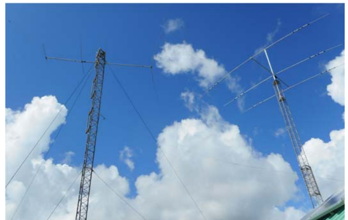
Part of the NP2X antenna farm in the Virgin Islands. Now just which of these Yagis went through a Category 5 hurricane with winds estimated at more than 200 mph? (H. Ward Silver, NØAX, photo)
