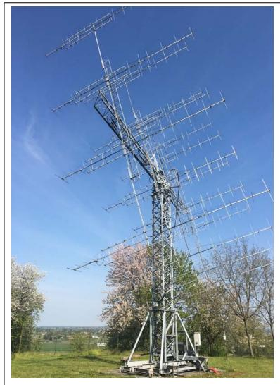
I2FAK's 144 MHz array: 16x19-element Log-Loop-Yagis in H plane, plus 16x6-element Yagis in V plane, with adaptive polarization on Receive. [Franco Giorgi, I2FAK, photo]
