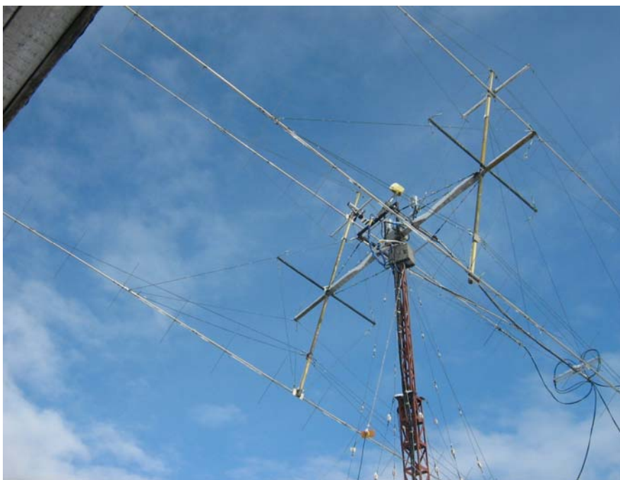
Sergey, RX1AS, showing how his 144 MHz Yagi array it is very well guyed for stability [Sergey Spiridonov, RX1AS, photo]
