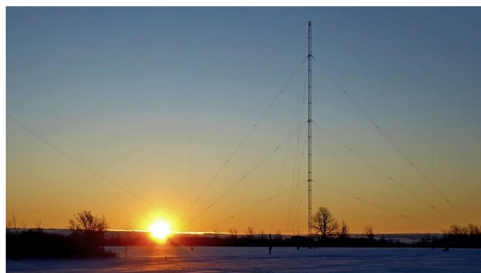
Sunrise greets the VE3EJ transmitting antenna. The 130-foot tower serves as the driven element and top-loaded vertical wires hanging from it can be configured as directors or reflectors, giving John a 3-element vertical Yagi in 4 switchable directions plus an omnidirectional mode. (Photo courtesy of John Sluymer, VE3EJ)
