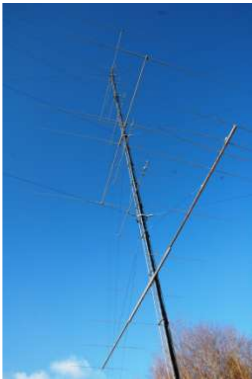
Tower No 1 at WW1WW supports a 4-over-4 OWA for 40, and five 5 element LFA-over-9 elements LFA on 10. (WW1WW photo)
