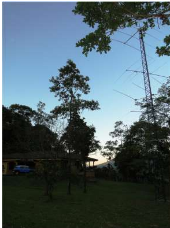
The T15W QTH: The 80 foot tower supports an M2 log periodic at the top, 10 and 15 meter stacks and a SteppIR — all bolted to the sides. The tall tree supported one corner of a 160 meter loop. (T15W Team Photo)
