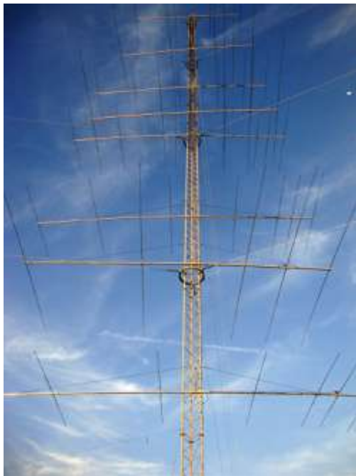
The No. 1 200-foot rotating tower of Rohn 65 at K4XS supports 5 element stacks for 20 meters at 200, 150, 100 and 50 feet and 7 element stacks for 10 meters at 120, 90, 60 and 30. (Photo by K4XS)
