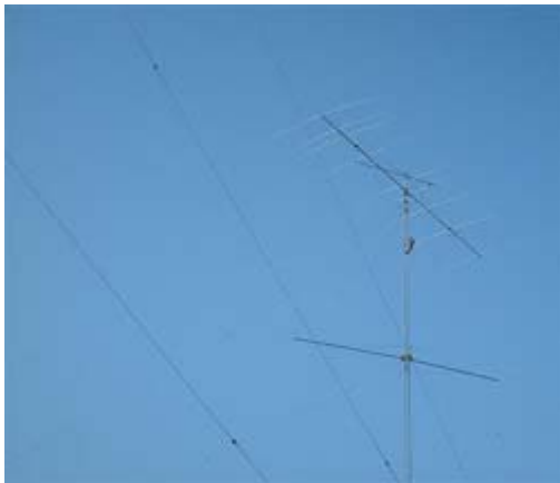
Check out the new 20 meter beam at M/M winner NQ4I . The antenna is 8 elements on a 86 foot boom at the top of Rick's 185 foot Rohn 55 tower. See www.nq4i.com for more information on the NQ4I station.
