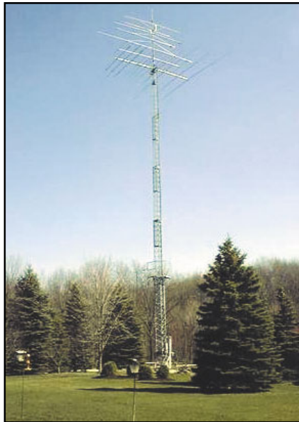
All VHF/UHF bands through 2304 are covered on this tower at N2BJ in Illinois.
