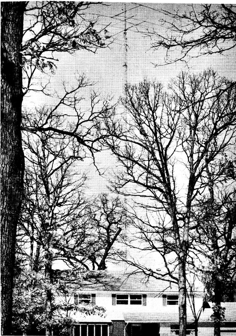
Hidden in the trees around the W0AIH/9 estate are four slopers, an extended Zepp at 120 feet and a 145-foot vertical, in addition to the Yagis at the top of the tower.
