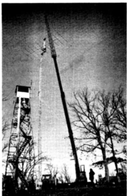
Logistics and teamwork are the name of the game for the Mecklenburg ARS. Shown are the fire-watch tower, 60-foot tower, and the 110-foot crane used as antenna supports. W4BFB/4 multiop effort netted 391 QSOs for 20k points to lead the Roanoke division for multiops.
