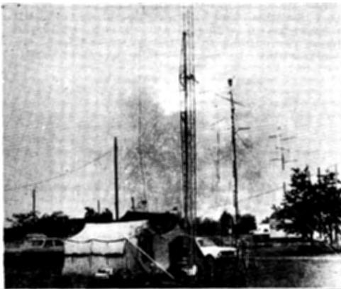
Over 100 of this year's entries were multiops. Here's W3CCX/3, the Mt. Airy VHF Radio Club, operating from Bucks Co. in Eastern Pennsylvania. Pictured above are their towers holding the 50, 144 and 220 MHz antennas while to the right, the 432, 1296 and 2300 MHz tent and 6' parabolic dish.
