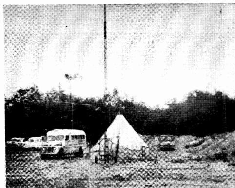
The Western Pennsylvania Section has always been tough for stations along the Eastern Seaboard, but this was remedied in the September Party by W3SDZ/3, atop Rauchtown Mtn. The most easterly high point in the section saw two towers, 60 and 70 feet high, erected for the occasion by K3SBQ, K3SHY and W3SDZ. A 7.5-kw. generator supplied power, and gear was housed in a converted school bus and a commercial radio mobile news cruiser. K3SHY at the mike.
