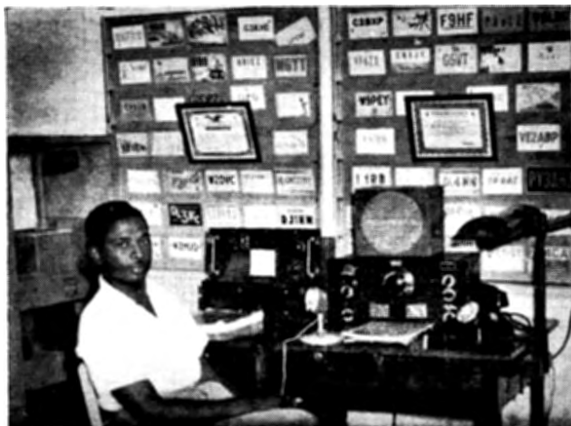
South American phone leader VP3HAG got 704 QSOs and 135,040 points with parallel 807s and dipoles but has a three-band quad ready for the '59 doings.
