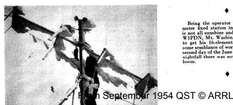
Being the operator of the highest 2meter fixed station in eastern America is not all sunshine and v.h.f. DX. Here W1PDN, Mt. Washington, N. H., tries to get his 16-element array back into some semblance of working order for the second day of the June V.H.F. Party. By nightfall there was nothing left but the boom.
